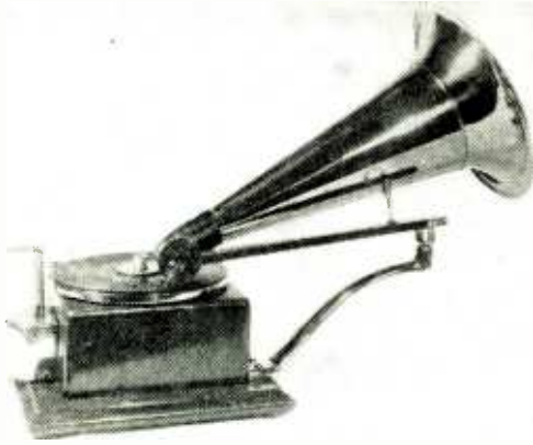
1897 needle-using disc gramophone
